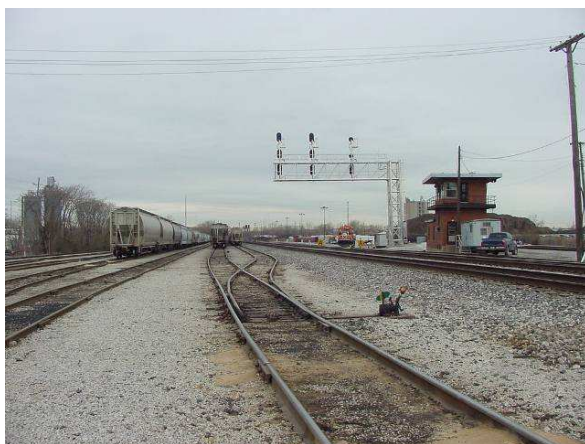
New signal bridge along the IHB in Summit, IL
