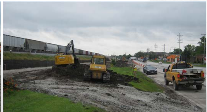
Excavation for construction of swale to Bensenville Creek
