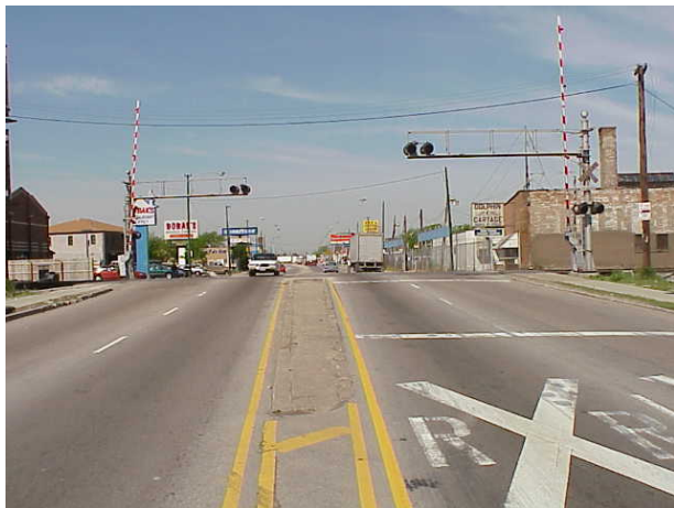
View facing Southwest on Archer Avenue
