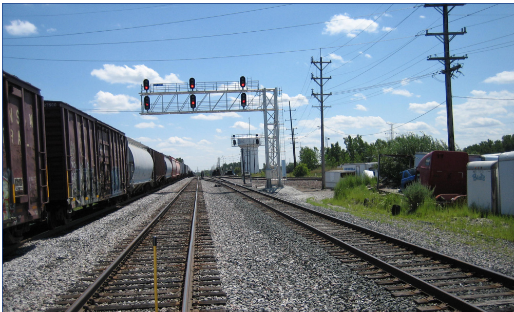
Thornton Junction Signal Bungalow and Cantilever
