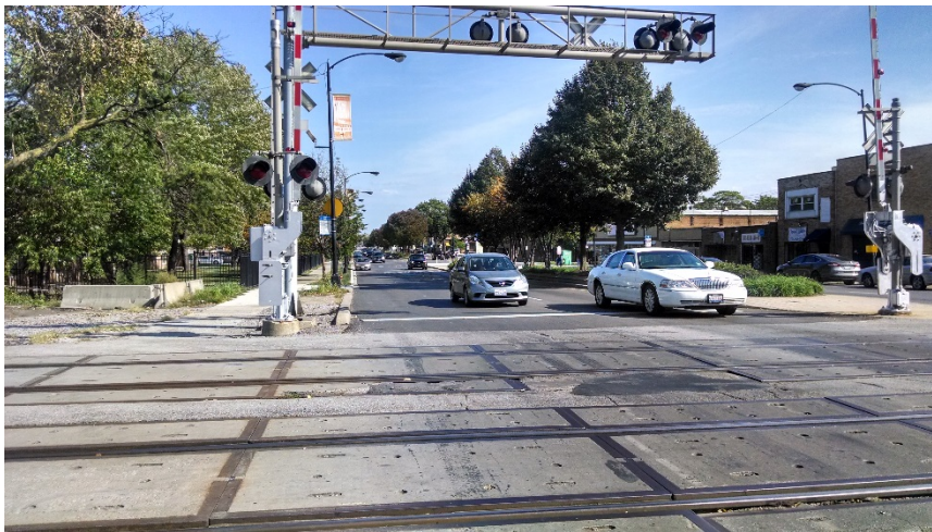
Figure 4.3 GS21a Existing Conditions
